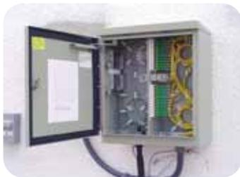
cable stubs so that the unit is quickly connected to the plant. The outdoor FDT may be pre-wired with pigtails on the drop side so that individual drops routed into the unit can be spliced to the connectorized pigtails. The unit accommodates a variety of OSP cable types via sealed grommet entry. Cables are secured with standard grip clamps to provide the required pull out strength. The enclosure provides grounding for metallic members and for the cabinet.
